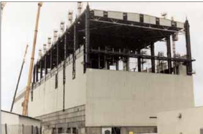
Above: roof at start of lift, single jacks mounted on each column extension. Two power packs, one on each side of the roof, controls the eighteen jacks split into two sets of nine.
