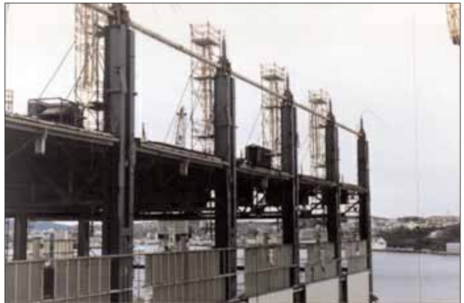
Above: roof at start of lift, single jacks mounted on each column extension. Two power packs, one on each side of the roof, controls the eighteen jacks split into two sets of nine.
