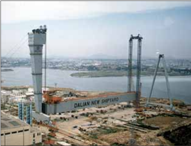
Below: Jacking system at top of completed pier leg performs lift with jacks mounted on relocated tower system at shear leg end. Below: completion of the pier leg 'chain lift'.
