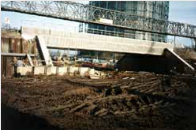
Above: The bridge in final position.
