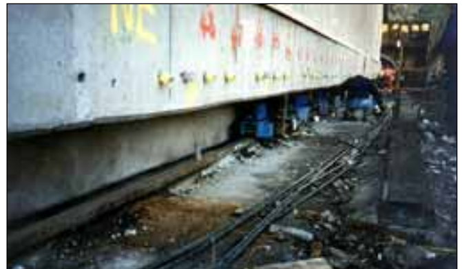
Above and Below: The vertical jacking facility provides a hydro-cushion support and controls final positioning.
