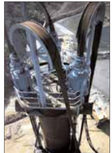
Above: Jack cluster at the top of a lifting tower.
