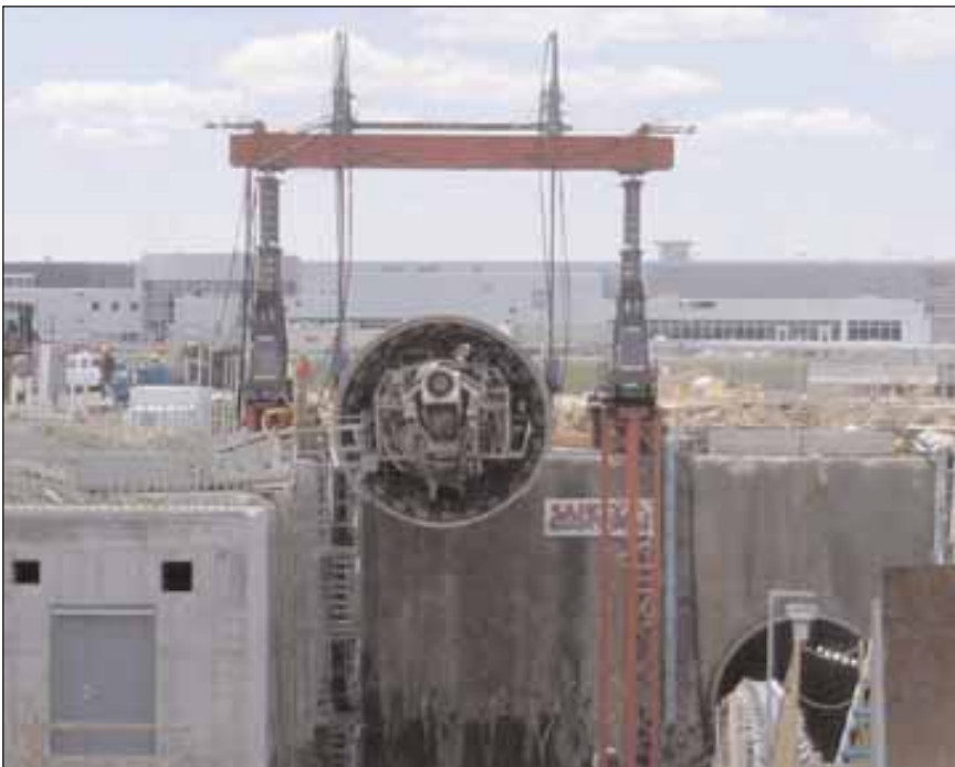
Left: North portal - Lift system in action, TBM half way.
