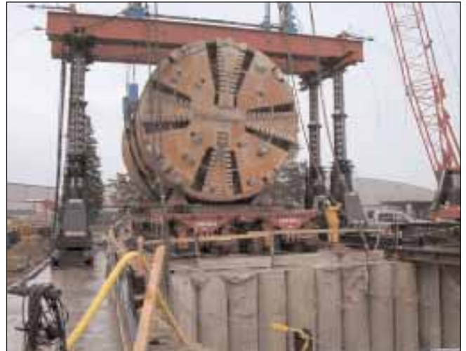
Above: South portal placing on to SPMT's
