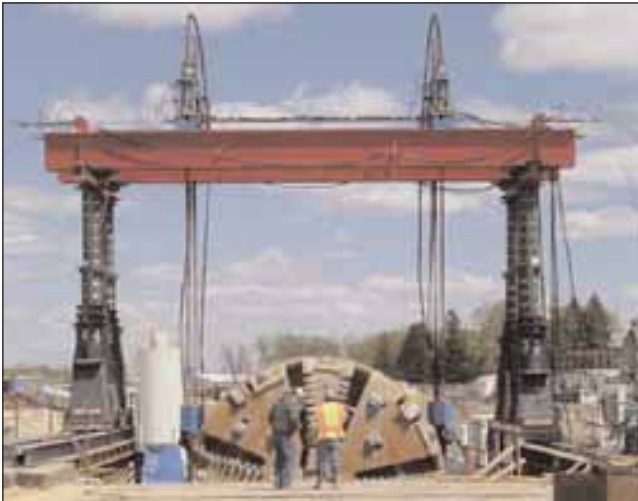
Above: TBM appearing, taken at ground level.
