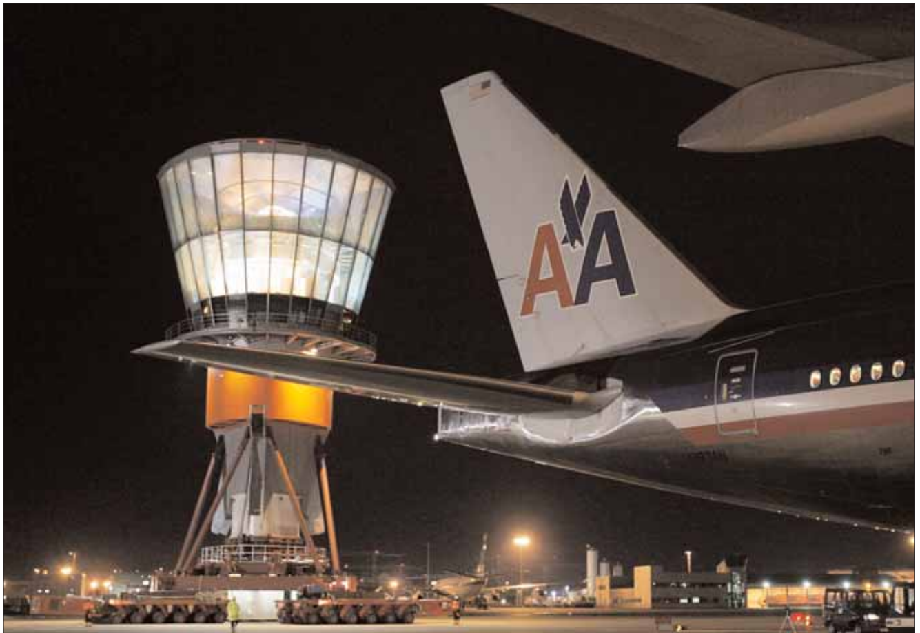
Above: Cab being transported overnight by three SPMTs
