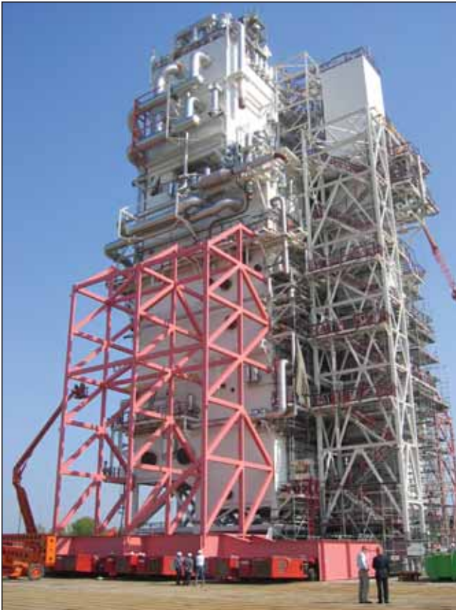
Above: Cold box prior to loadout
