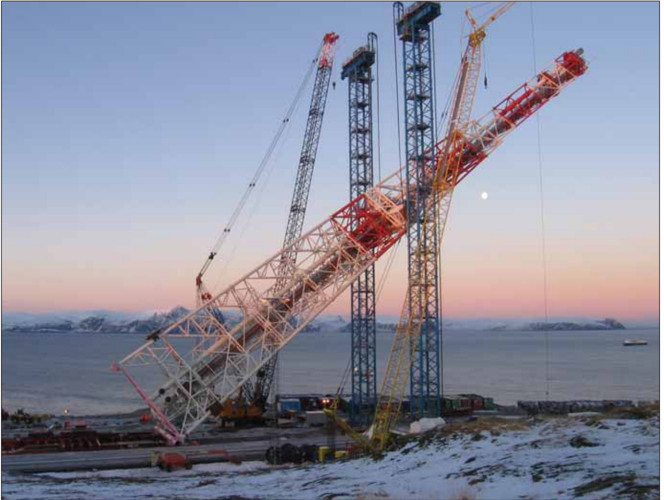
Above: Another photo of the spectacular erection of the flare tower.
