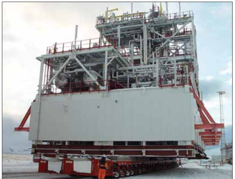
Below: A photo of a 900 tonne module being transported using SPMTs
