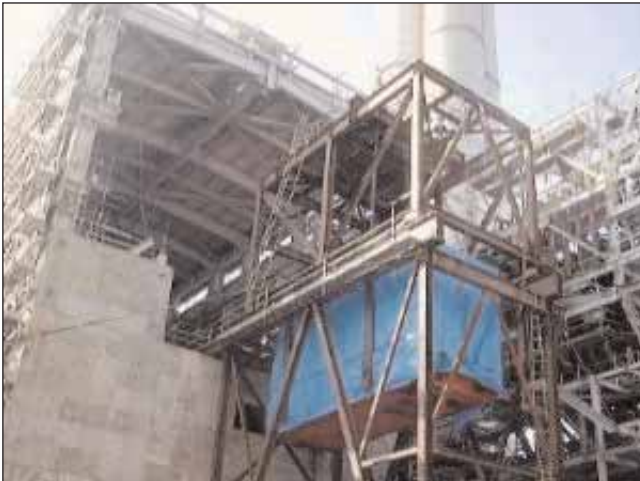
Above: The generator unit being lifted inside the travelling frame.
