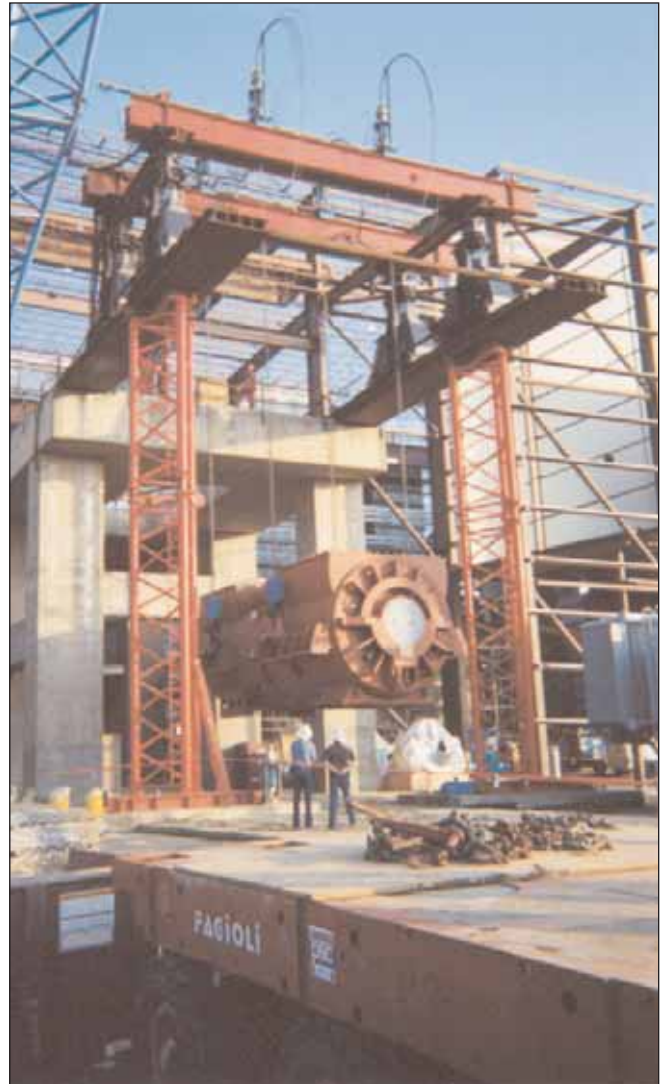
Above: Lift in progress
