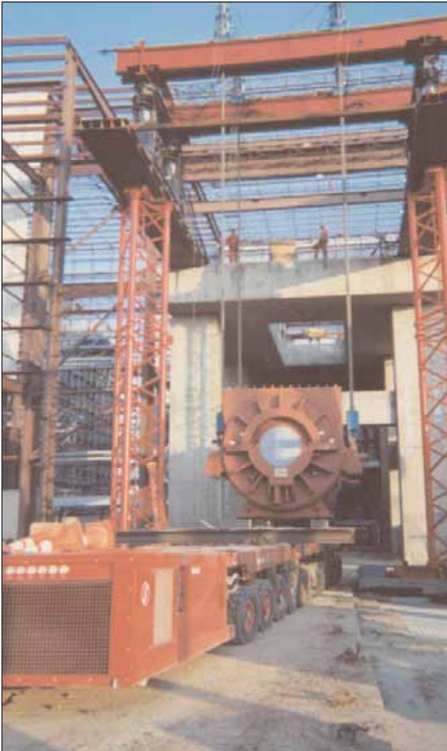
Above: Steam turbine generator just lifted off the transporter
