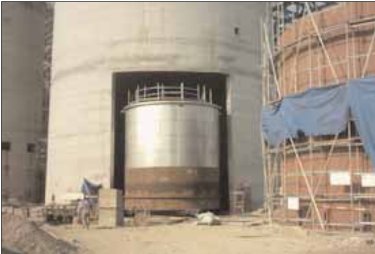
Above: The first can delivered to site to be lifted
