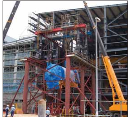
Above: Generator weighing 310 tonnes being lifted by the same lifting system.
