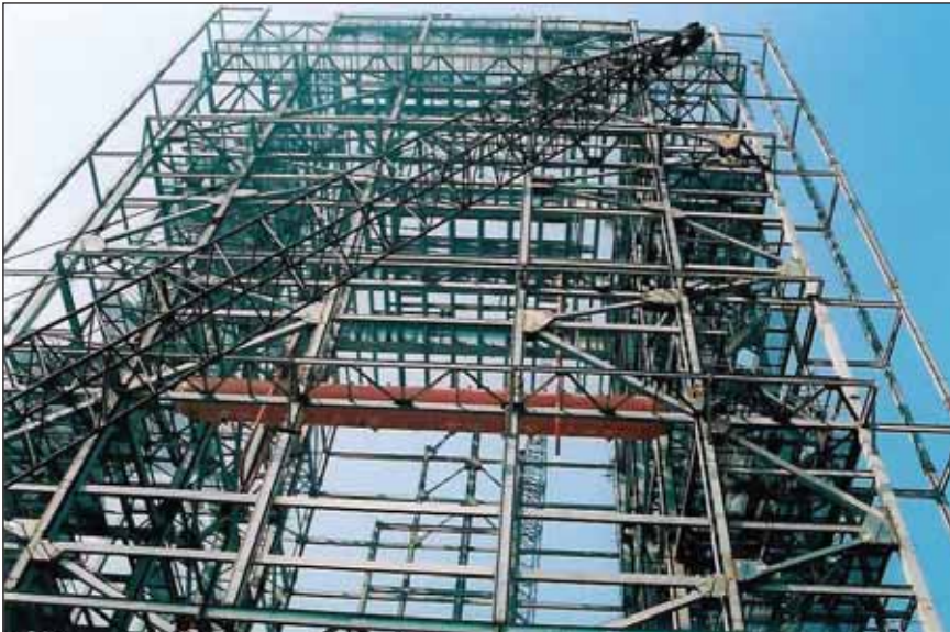
Above: View of lifting of boiler drum
