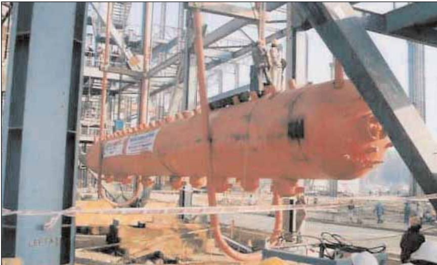
Below: Initial view of boiler drum
