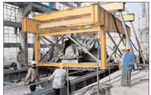
Top: Lifting of generator Directly above: View of L15 pulling jack Below: Skidding of turbine
