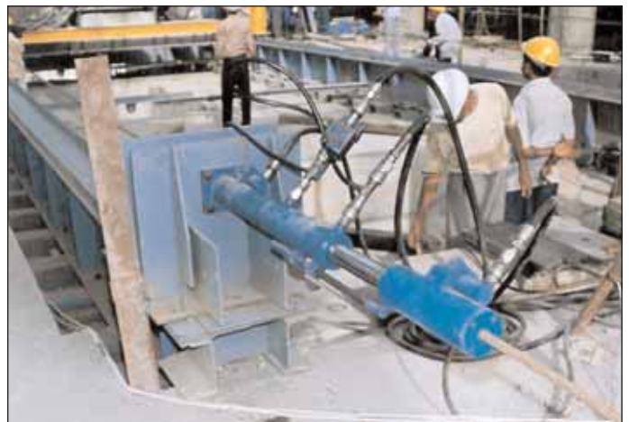
Top: Lifting of generator Directly above: View of L15 pulling jack Below: Skidding of turbine
