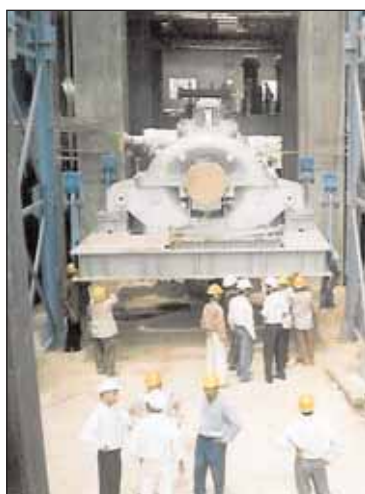
Above left to right: Turbine lift and generator lift
