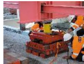
Climbing jacks are used to raise and lower heavy loads. Range from 200 to 600 ton. This kind of raising and lowering operations is carried out in steps of 10 cm
