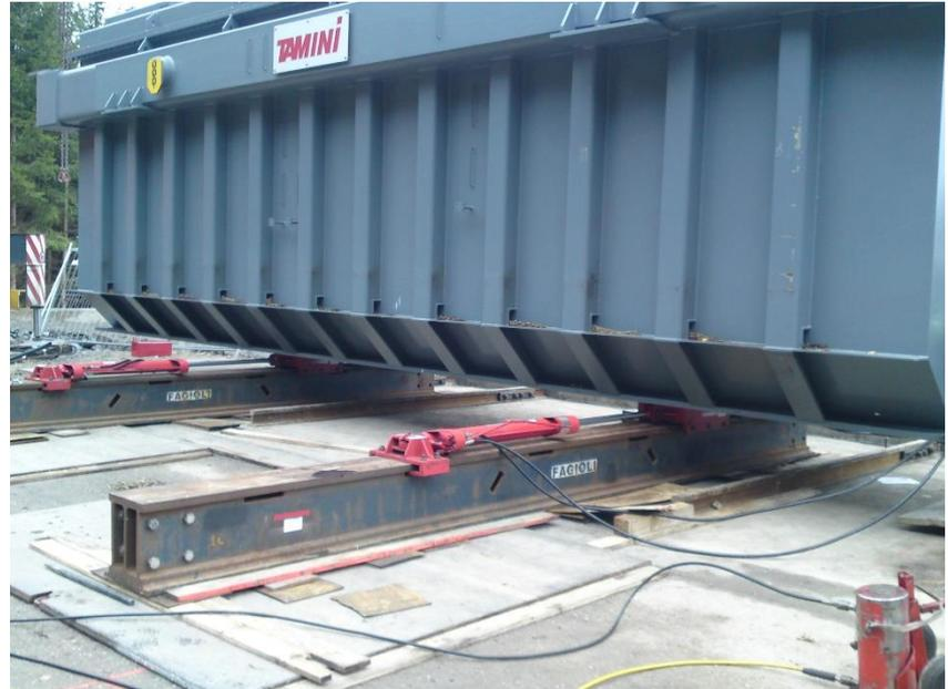
Once arrived at destination Fagioli lifted the trafo with the screw jacks in order to allow the trailer to be removed. The item was skidded with the rollers in order to align it to the tracks specially made on the foundations. Once in position, the trafo was hoisted with the hydraulic jacks allowing the Fagioli operators to place the wheels under the transformer (after the skidding beams removal). Eventually, the transformer was pushed onto tracks to its final position with winches
