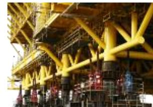
Fagioli patented Push-up System has been designed to provide impressive hoisting operations such as offshore decks and platform
