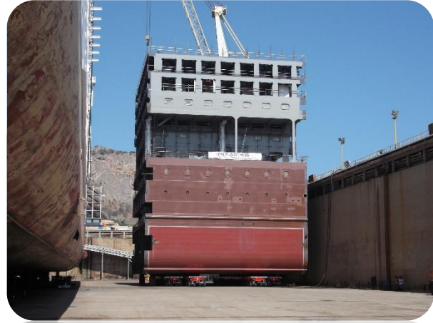
On top: Section positioning by SPMTs
