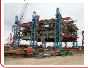
Sime Sembawang Engineering contracted Fagioli PSC Asia to carry out the lifting of the Yo-Ho EPC2 deck. The 740 tonne upper deck section was constructed at the lift location and lifted using 6 of Fagioli PSC's 24 metre high square format towers and 12 Strand Jacks. This allowed the installation and mating of the main deck section.
