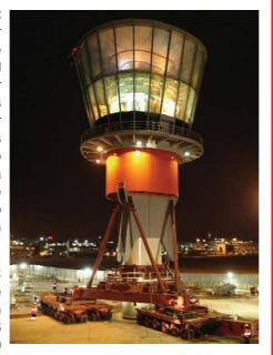
Strand Jacks. The top section of the VCR will be lifted 12 metres at a time to install underneath  $4 \times 12$  metre steel sections.
