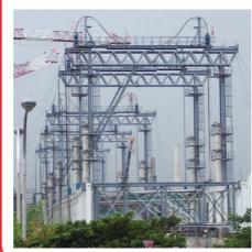
To cope with the increasing amount of passengers coming in and out of Singapore and the next generation aircraft A380, the new terminal 3 was built at Changi Airport. Fagioli PSC Asia was awarded the contract to carry out the lifting for 10 bays of roof trusses. Each roof truss weighed 610 tonnes with a width of 15 metres and a span of 220 metres.
