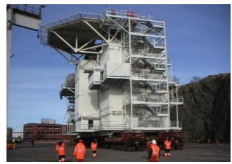
Three weeks later Fagioli SpA carried out another loadout of a 1,200 tonne BP Mad Dog module (above) destined for the Gulf of Mexico. This project was similar to the previous loadout as the site move also required a sharp 90 degree turn on leaving the fabrication hall and then a 180 degree 'carousal' turn to ensure the L.Q. Helideck would not clash with the ships starboard side crane pedestals.
