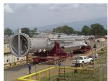
Fagioli PSC USA were contracted by Marathon to provide transportation of heavy pieces from the port to their refinery in Malabo, Equatorial Guinea. The project required 24 lines of SPMTs and a hydraulic gantry as well as 2 - 4 men on site for approximately 1½ years to transport and install refinery processing equipment including reactor vessels up to 300 tons. Fagioli received letters commending the crew, staff and company for a successful operation.
