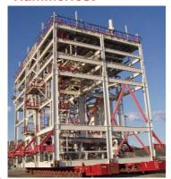
Fagioli SpA carried out the transport, lift and installation of 100 modules for a new LNG plant under construction on Melkoja Island off the Northern coast of Norway. The project is to be carried out through the warmer months of 2004 and 2005 due to extreme weather conditions.
