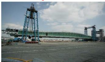
Fagioli PSC were sub-contracted by Watson Steel to transport and erect the connector bridge to the new pier at Gatwick Airport.
