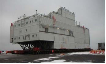
Fagioli SpA performed the loadout of two living quarter modules in Gothenburg, Sweden for Pharmadule Emtunga. The first loadout was for a 2,200 tonne Kristen Living Quarters (above). The loadout was performed using 138 axles of SPMTs to move the structure 500m from the fabrication hall to the loadout quay. The site move was particularly challenging as the exit from the hall required a 90 degree turn with as little as 1m clearance on either side.
