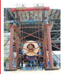
Fagioli PSC Asia was awarded the contract to install the gas turbines & generators for Tuas Power Station Block 3&4, Singapore. 150 tonnes of temporary structure was designed, supplied and erected by Fagioli PSC
