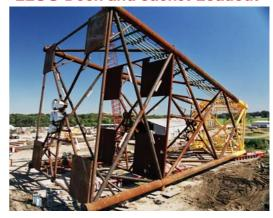
A deck and jacket were loaded out with SPMTs at Chet Morrison's Fabrication yard in Houma, Louisiana. Both pieces weighed about 700 tonnes. The jacket was moved from the yard area onto a barge using 10 meter long ramps also supplied by FPSC.
