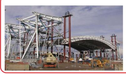
The new Terminal 5 main building at Heathrow Airport has a roof structure with a total weight of 18,000 tonnes. On completion this roof structure will be the largest single span building in the U.K., the total floor space occupying the equivalent of 50 football pitches.
