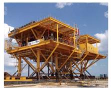
A 2,500 ton jacket loaded out over 450 feet in Corpus Christi, Texas. The combination of 4 x L180 Strand Jacks and an L4/35D power pack achieved pulling speeds up to 60 feet per hour. The
