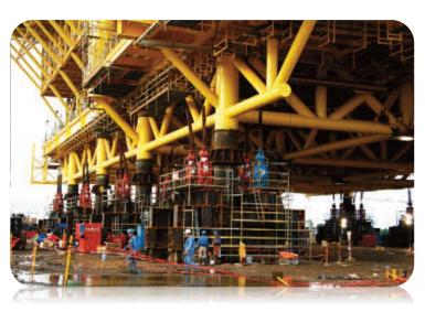
The Lifting Frame was made of two connected symmetrical items and by 4 Shear Keys, sliding above the frame. Each Shear-key operated by a couple of double—acting jacks, powered by a dedicated hydraulic system. The lift was carried out in five steps, 150 cm high each.
